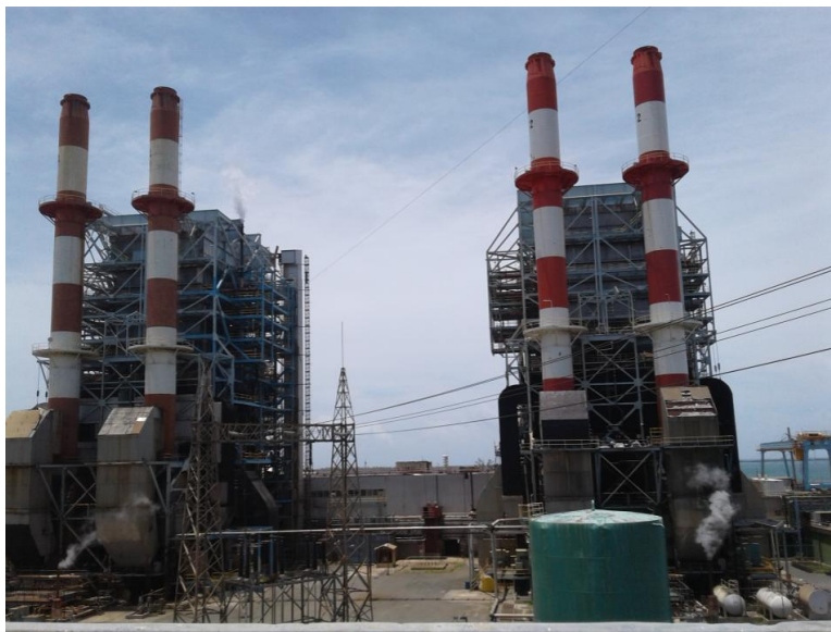
Figure 2. Oil-Fired Power Plant in Salinas, Puerto Rico, 2018
